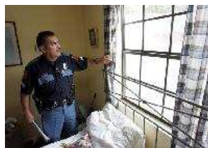
Officer Joe Milian inspects the windows for secondary locks. (Mark Lambie / El Paso Times)
